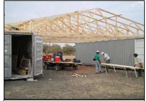
Setting Rafters on the Containers
