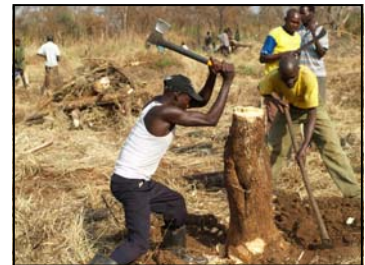
Clearing the Land
