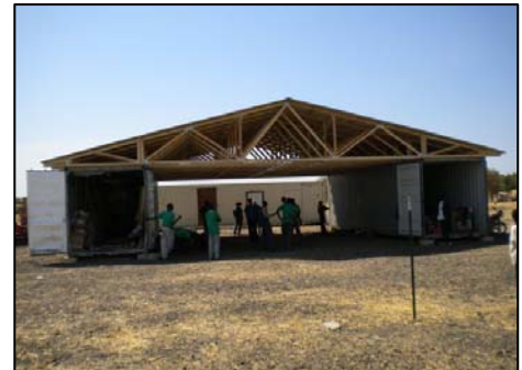
The Church Roof on the Container "Walls"
